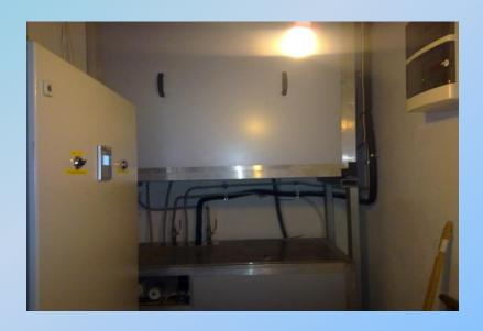
Technical room should be located up to 5 meters from the cave. It can even be placed on a higher level. It contains mostly device. Its dimensions should be at least 2,5 m x 2,0 m.
